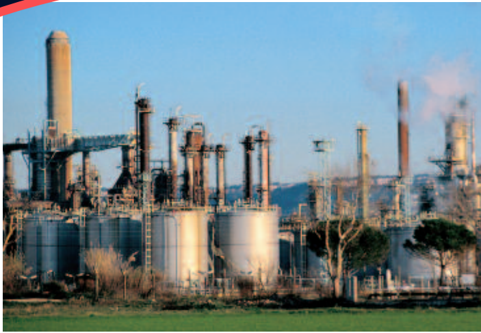
Petrochemical plant, 30 ha
